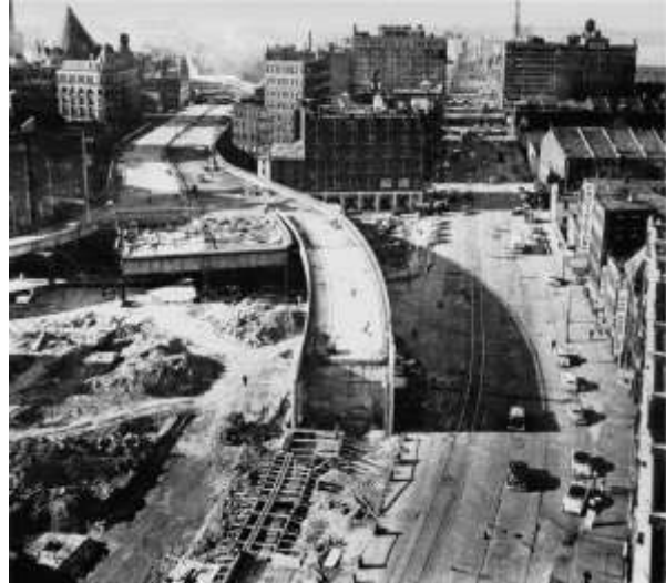
Construction of the Boston Central Artery around 1951, destroying the densely built inner city. https://hu.pinterest.com/pin/48906345925773502/
