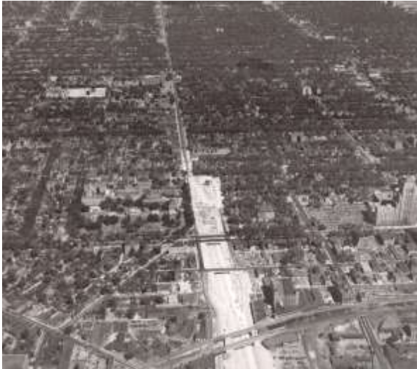
Detroit, construction of the first Expressway, 1949. https://skyscraperpage.com/forum/showthread.php?t=122541
