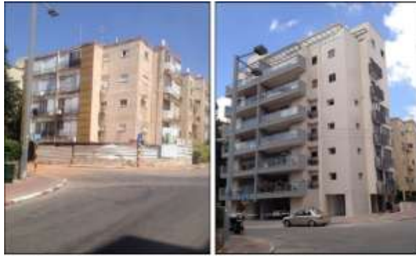
Figure 12: A condominium renovation project under National Outline Plan 38 (Tama 38) in Israel before (left) and after (right) renovation (Source: Hanani, 2015).
